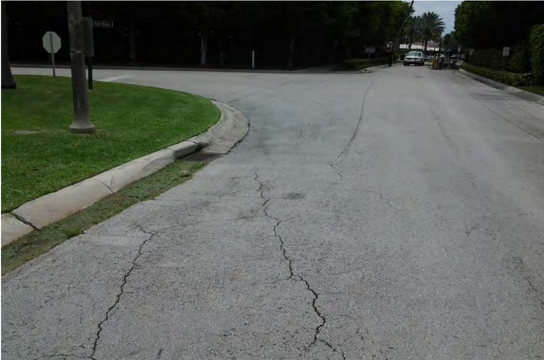
Photo 13 : Bal Bay Drive, road and curb failures, looking south.
