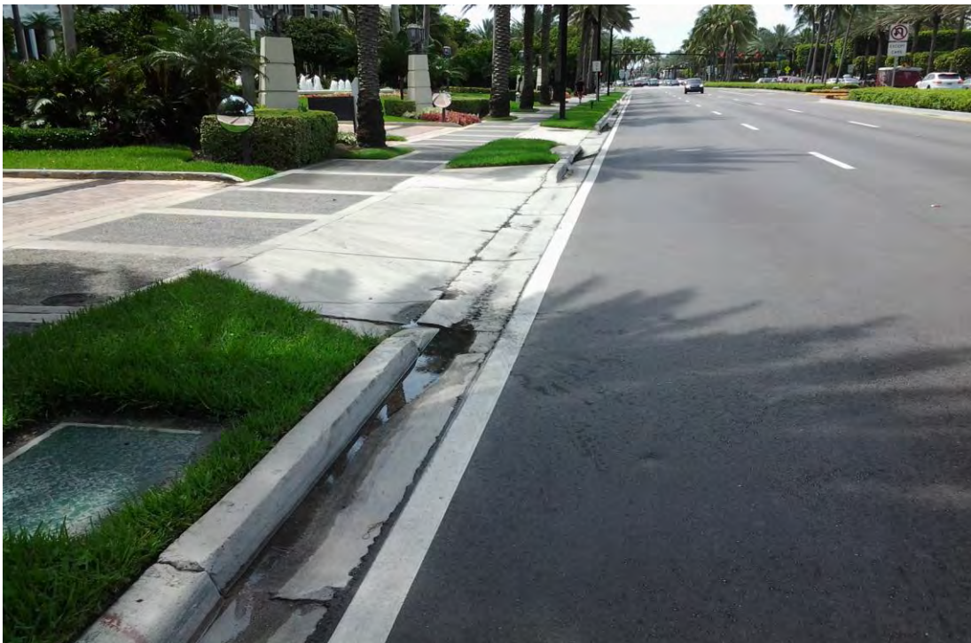
Photo 14 : Damaged curb and gutter at Bal Moral , looking south.
