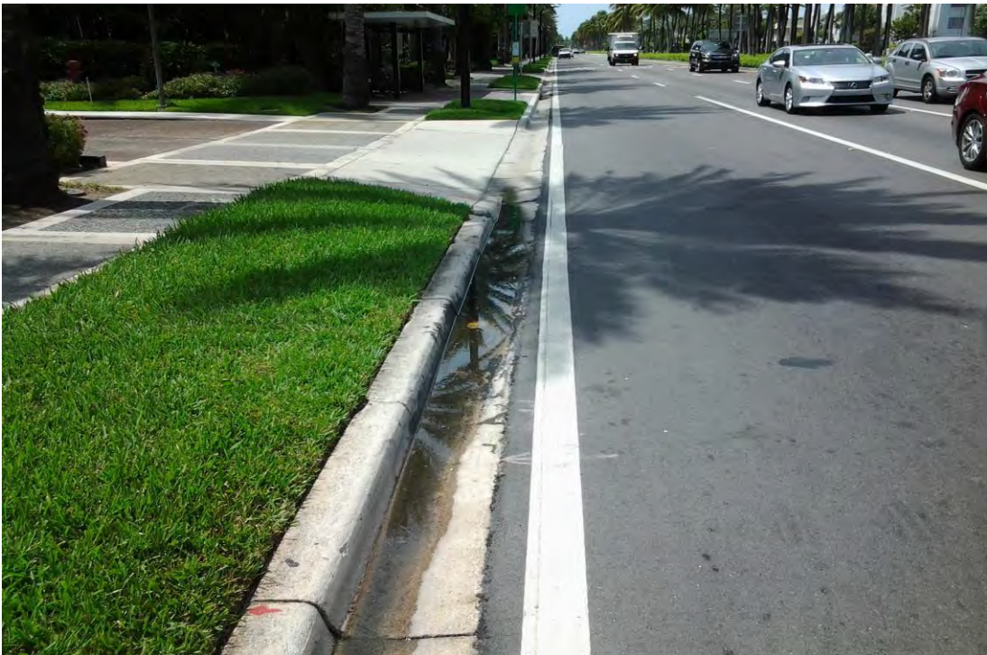
Photo 8 : Ponding in gutter on east side of Collins Ave., looking south.
