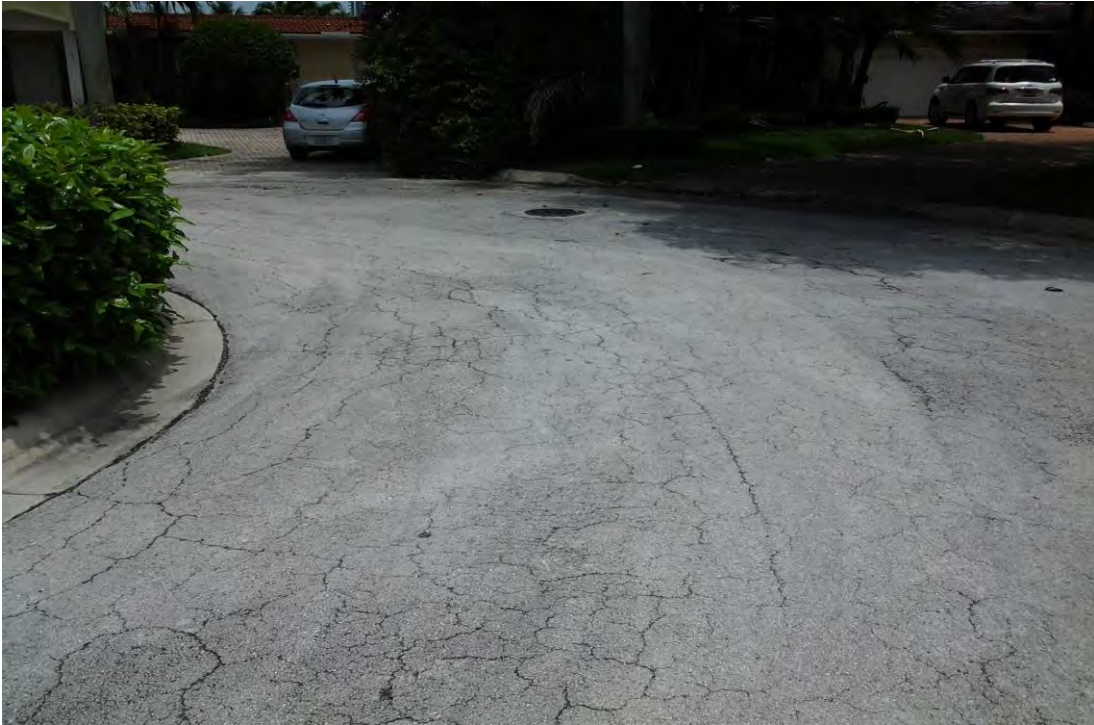
Photo 15 : Camden Court, road surface cracking, looking east.
