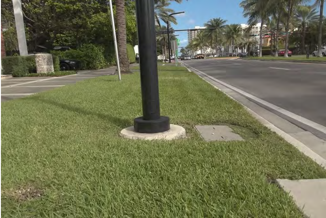
Photo 9 : Existing light pole pedestal and pull box in green area.
