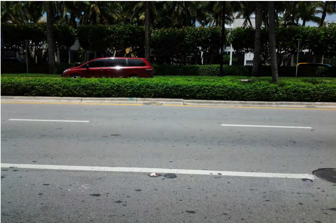
Photo 16 : Curb and Gutter settling in center median, looking west.
