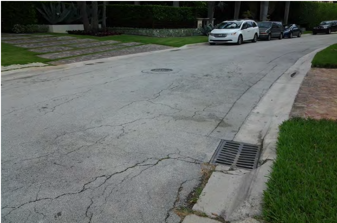
Photo 6 : Bal Bay Drive, road and curb settling, looking northeast.
