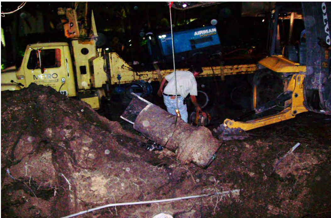
Photo 4: Sanitary Sewer Force Main repairs on Collins Avenue.
