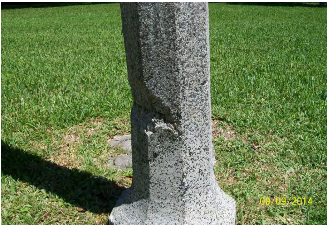
Photo 6: Damaged concrete pole base (152 Park Drive).
