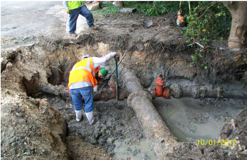
Photo 3: Thrust block removed in repair of leaking valves.
