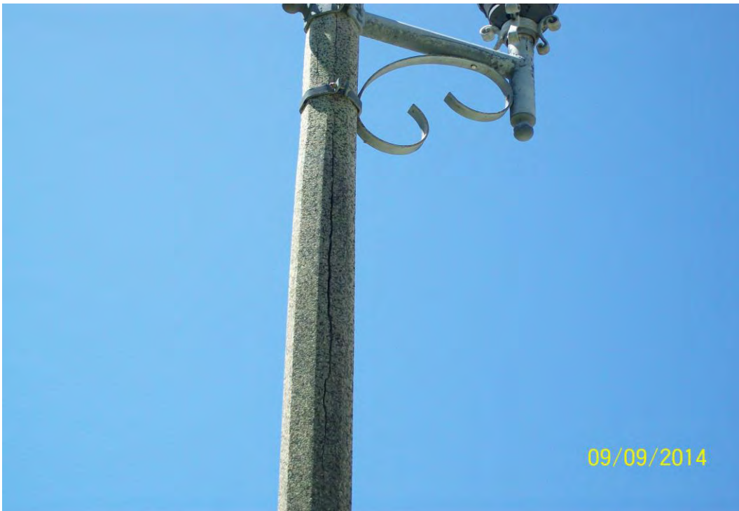
Photo 10: Longitudinal cracked concrete light pole (261 Bal Cross Drive).
