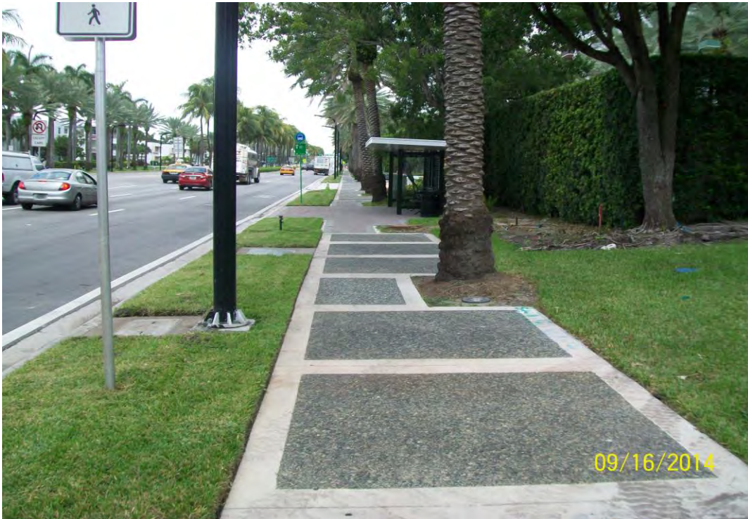
Photo 7: Existing light pole with missing base, looking north.
