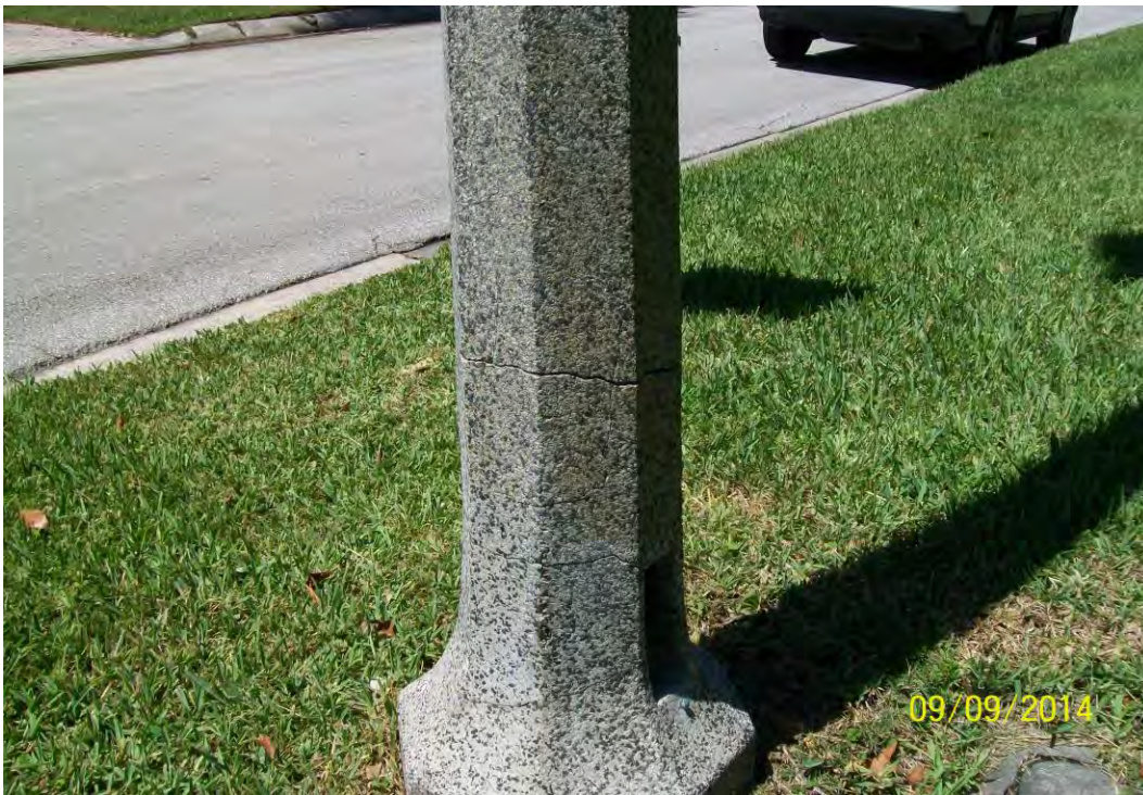
Photo 8: Cracked concrete pole base (261 Bal Cross Drive).
