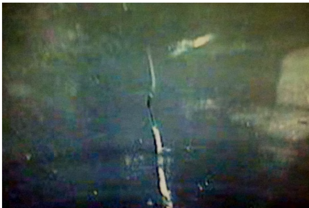
Photo 14: Longitudinal crack at top of stormwater pipe.
