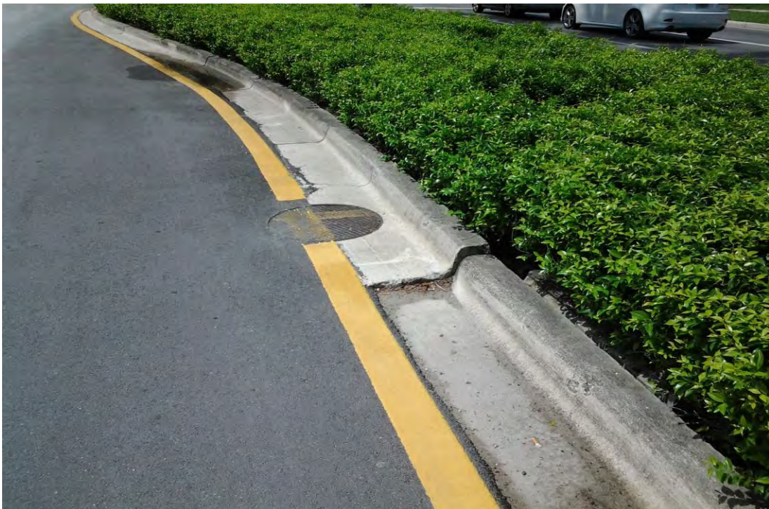
Photo 6 : Curb settling in northbound median, looking south.
