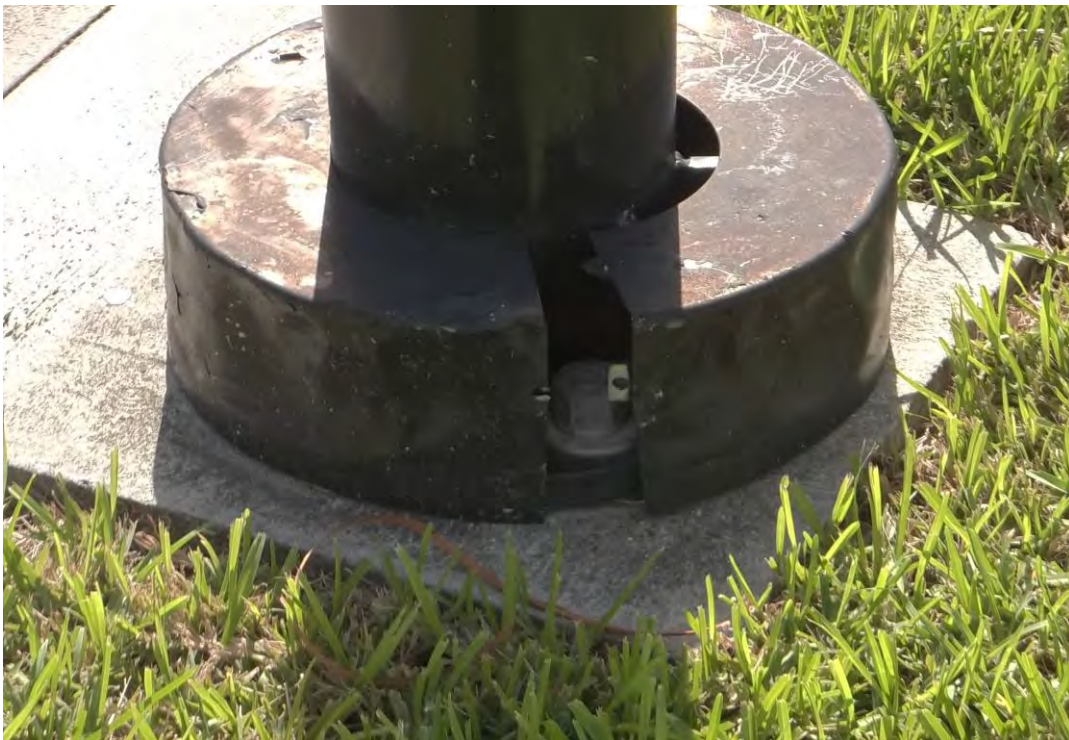
Photo 14: Existing damaged light pole base.
