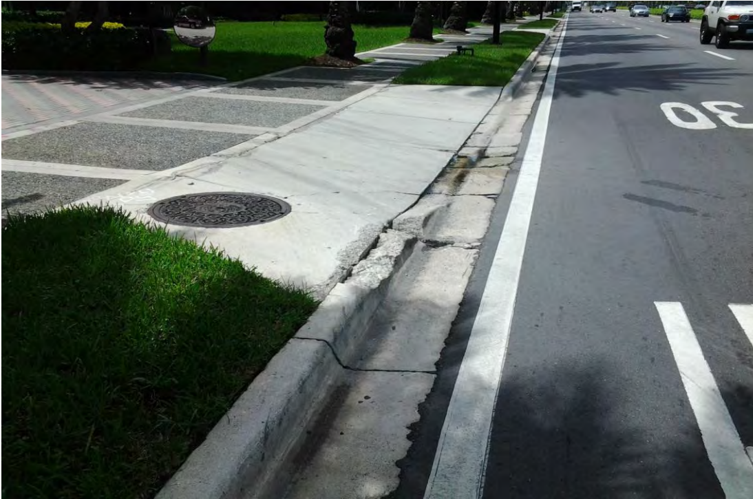
Photo 9 : Curb failures at 101 Bal Harbour , looking south.
