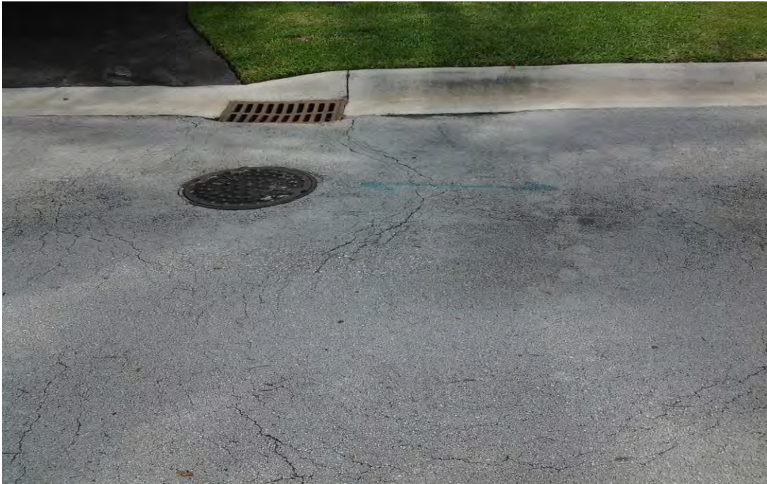
Photo 3 : Bal Cross Drive, road surface cracks, looking east.
