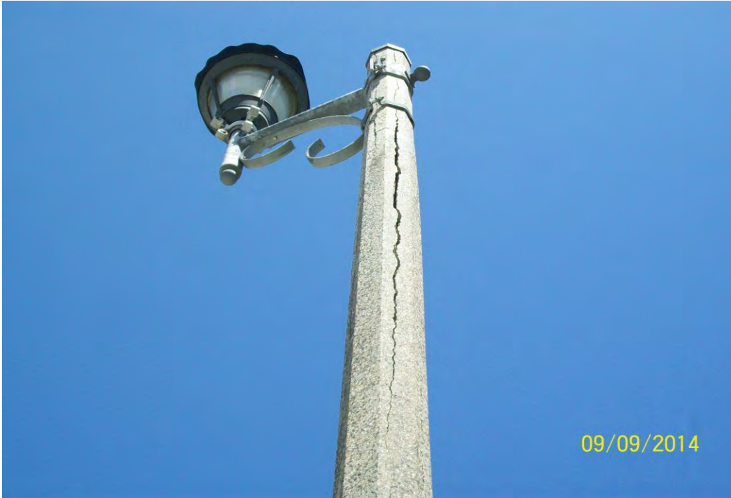
Photo 9: Cracked concrete light pole at Harbour Way East and Park Drive.
