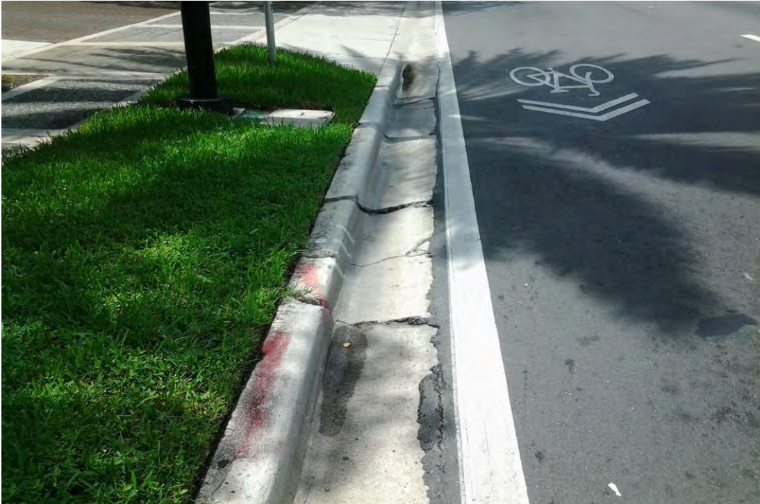
Photo 7 : Curb failures at Plaza of Bal Harbour , looking south.
