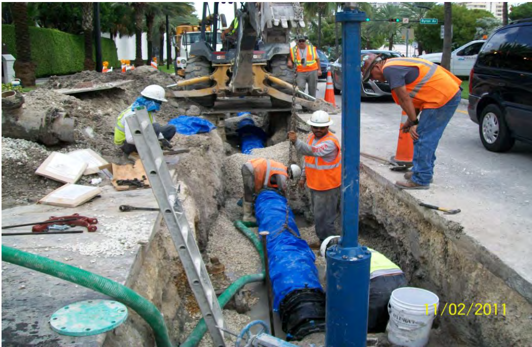
Photo 21 : Repaired 12" water main on 96 th Street.
