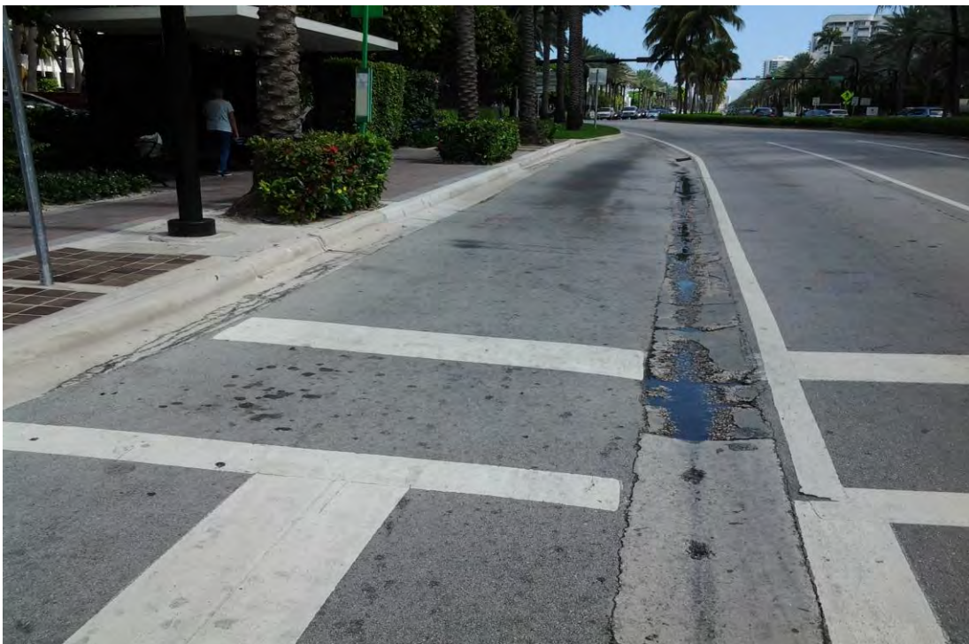
Photo 2 : Damaged concrete gutter at Shops Bus Stop, looking north.
