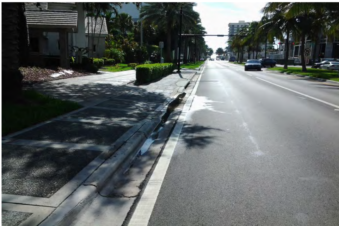
Photo 6 : Ponding in gutter on north side due to settling, looking east.
