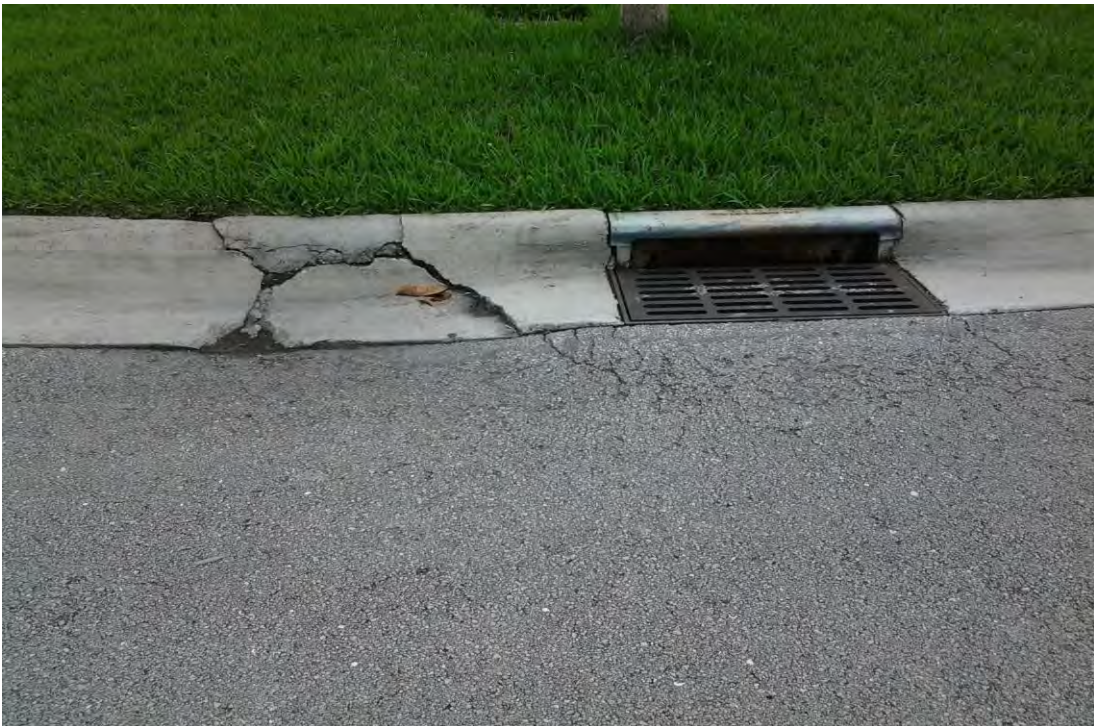
Photo 8 : Bal Bay Drive, curb failure, looking southeast.
