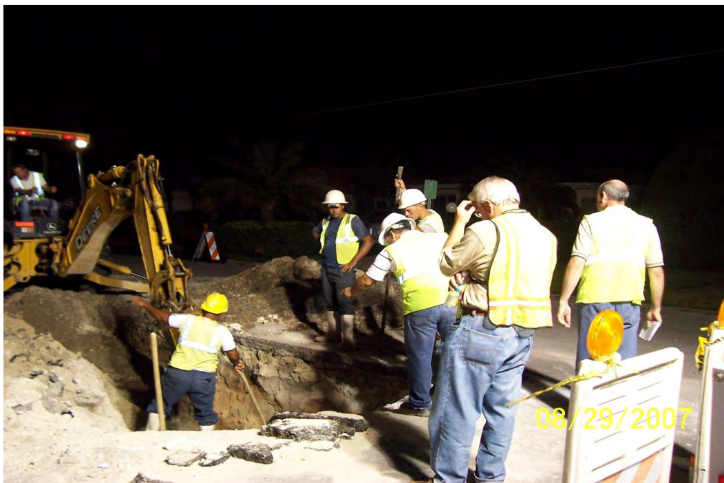
Photo 2 : Sanitary Sewer Force Main repairs on Byron Avenue.
