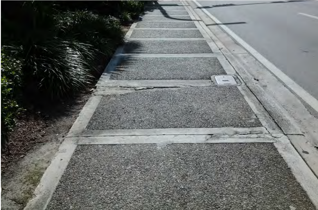
Photo 7 : Sidewalk cracking, north side of road, looking east.
