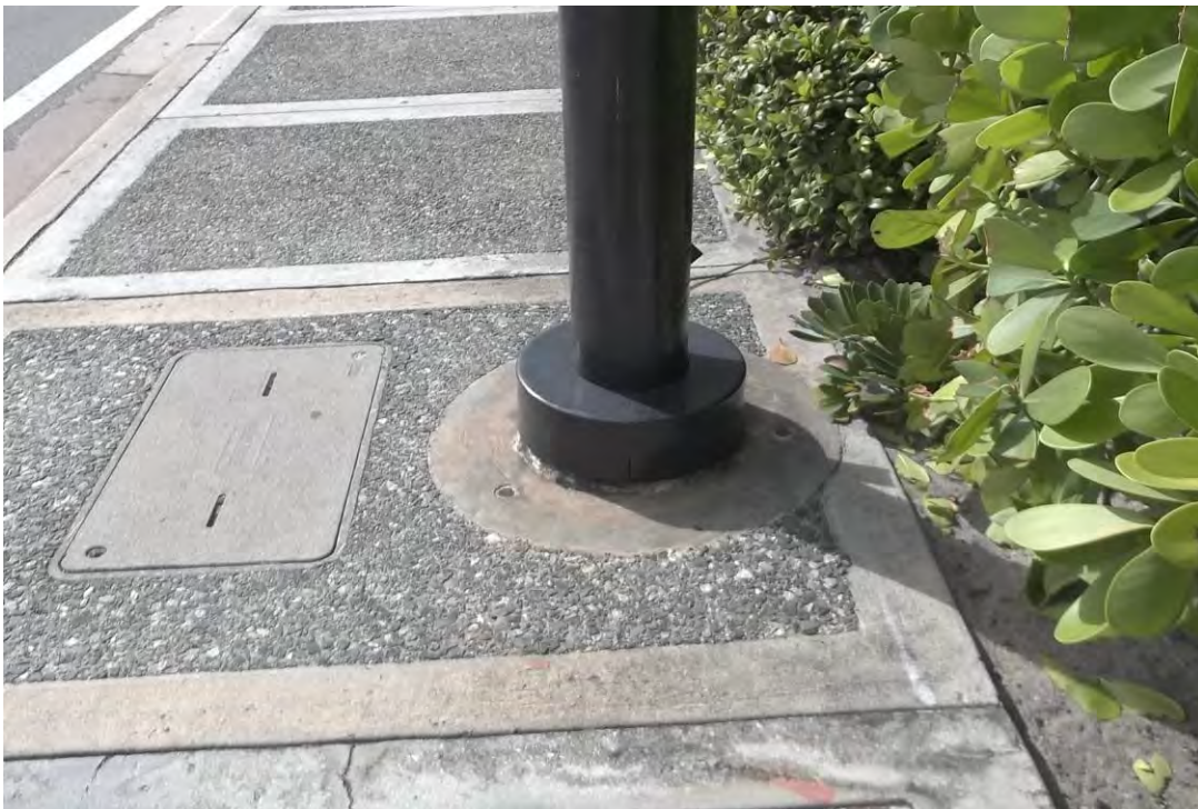
Photo 4: Existing light pole pedestal and pull box, located in sidewalk.
