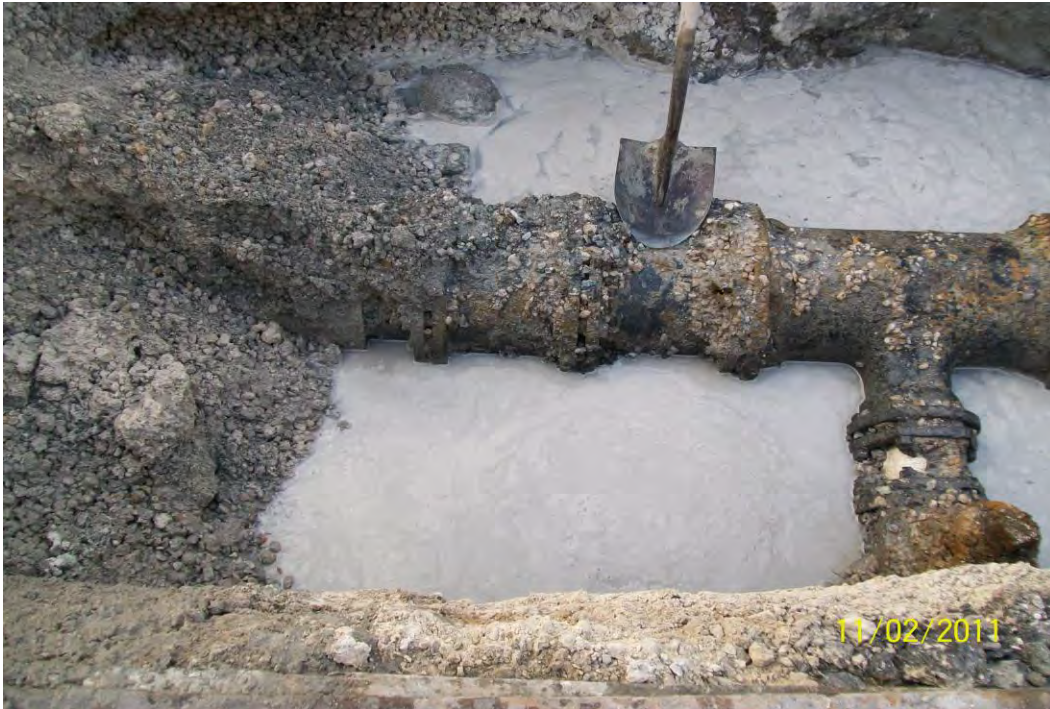
Photo 15 : Leaking water main pipe uncovered.
