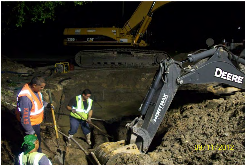
Photo 12: Night repair of water main on Park and Balfour Drive.
