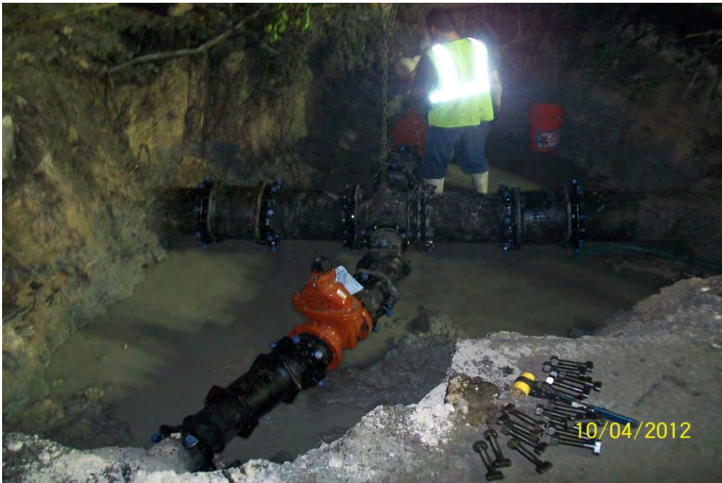
Photo 7: Installed emergency repair replacement pipe.
