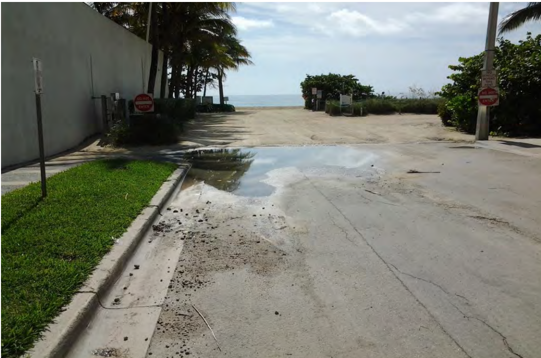
Photo 10 : Ponding at easternmost end of 96 th Street, looking east.
