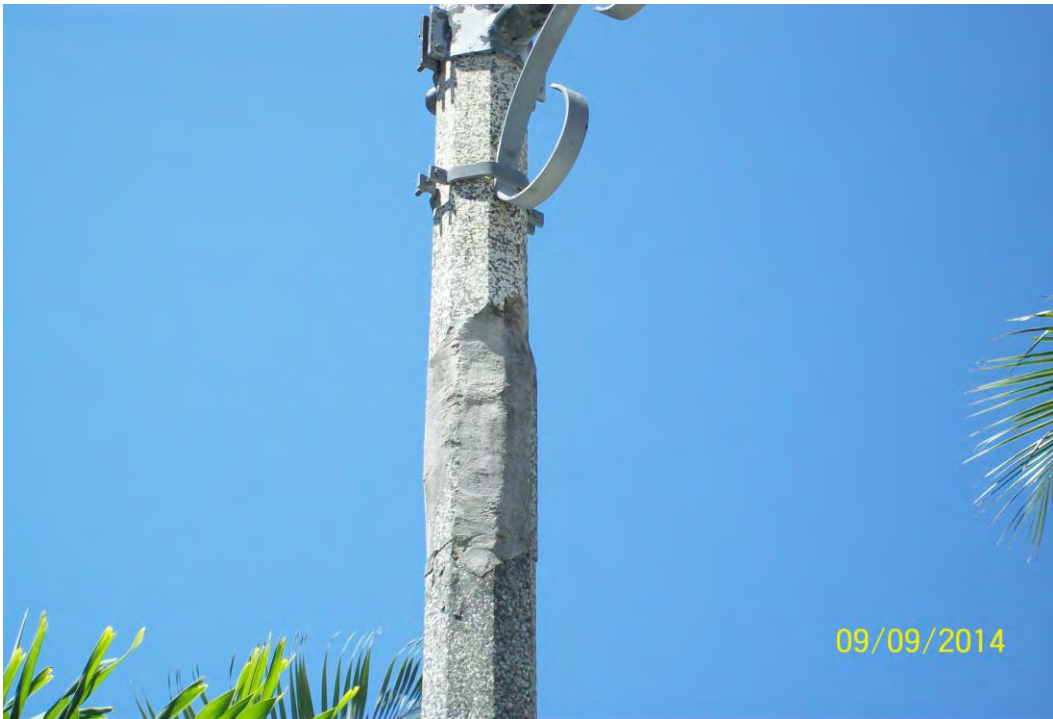
Photo 4: Repaired concrete light pole (126 Bal Cross Drive).
