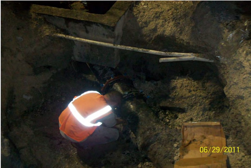
Photo 9: Sanitary Sewer Force Main repair on 96 th Street.
