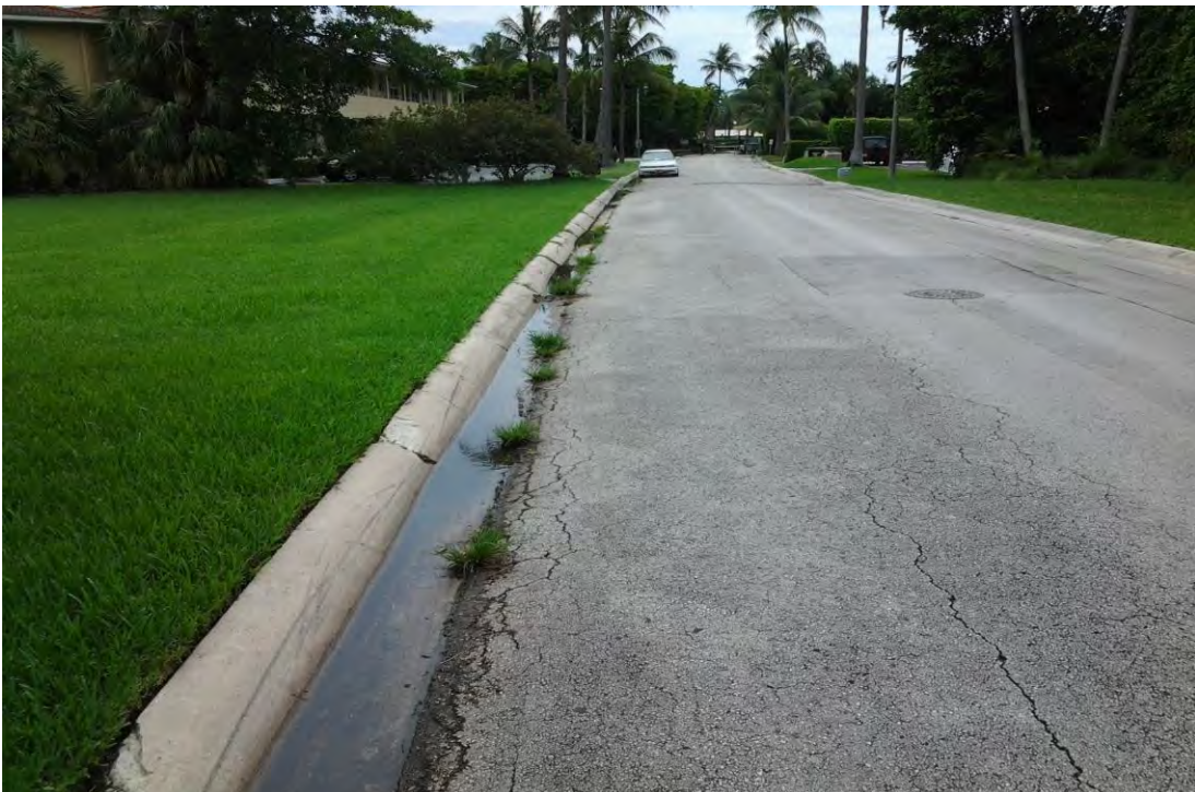
Photo 14 : Bal Bay Drive, curb settling and ponding, looking south.
