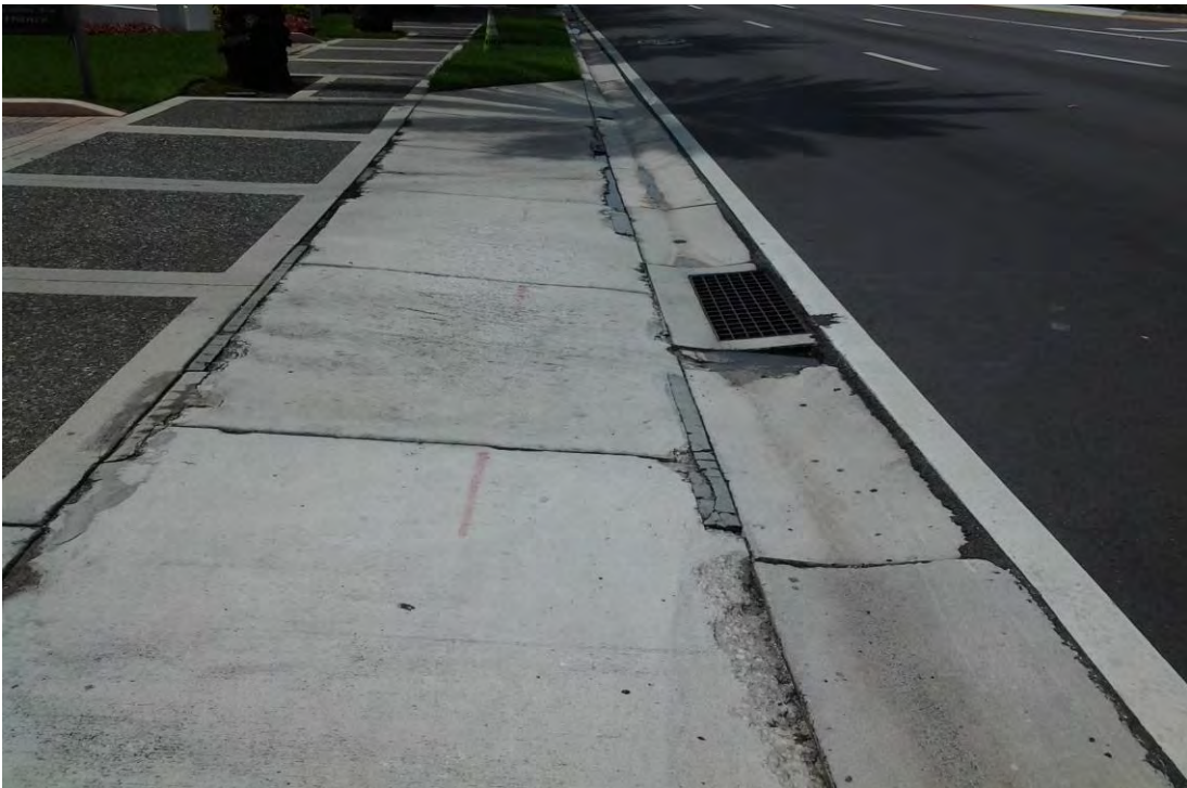
Photo 10 : Driveway approach damage at Seaview Hotel , looking south.
