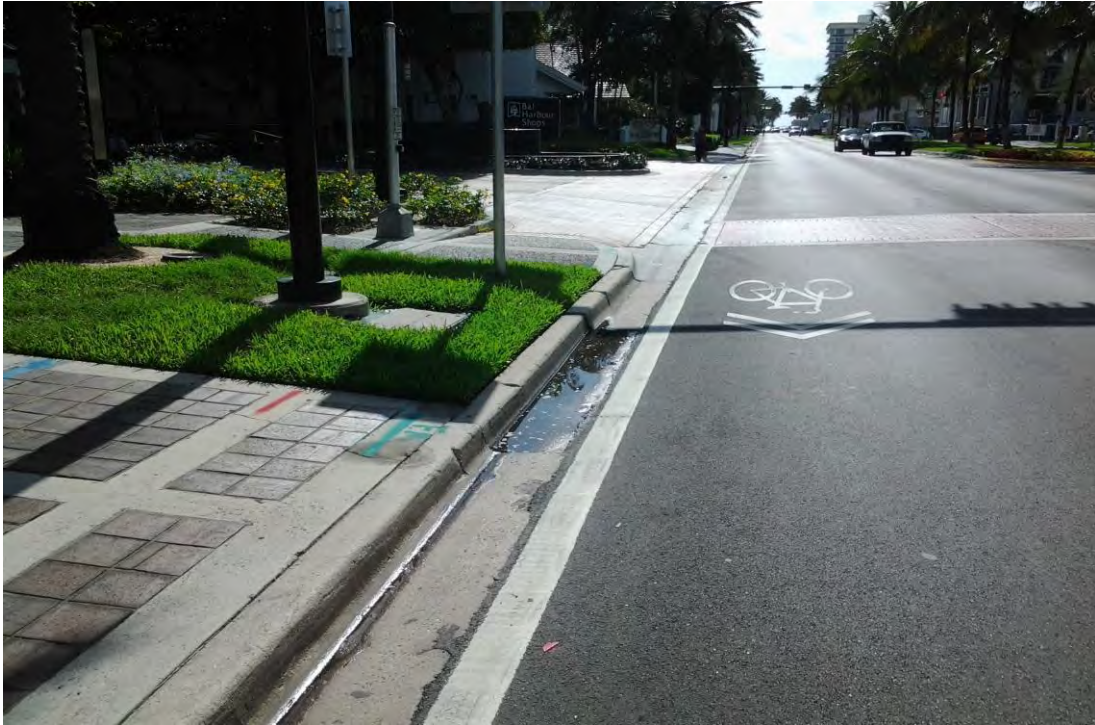
Photo 1 : 96 th Street, curb & gutter ponding, looking east.
