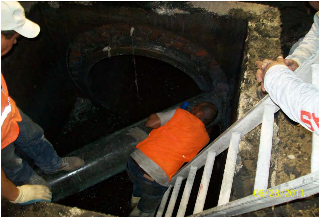
Photo 5: Sanitary Sewer Force Main repair on 96 th Street.
