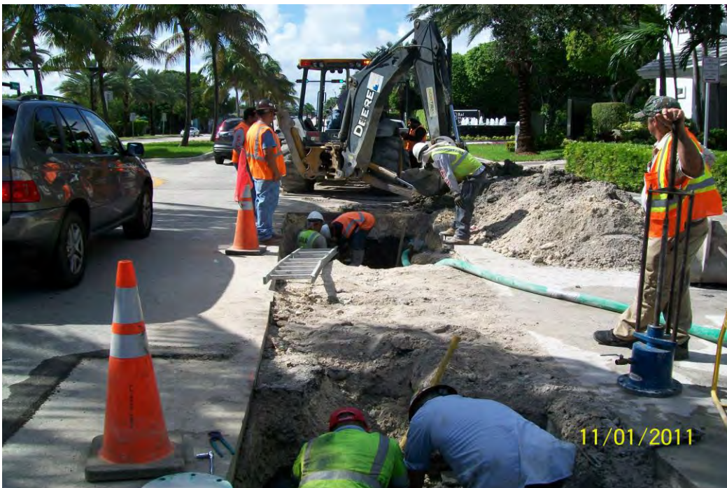
Photo 14 : Water main repair trench on north side of 96 th Street.
