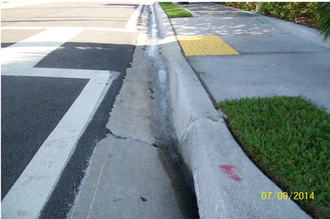
Photo 18 : Damaged gutter in front of Carlton Terrace , looking north.
