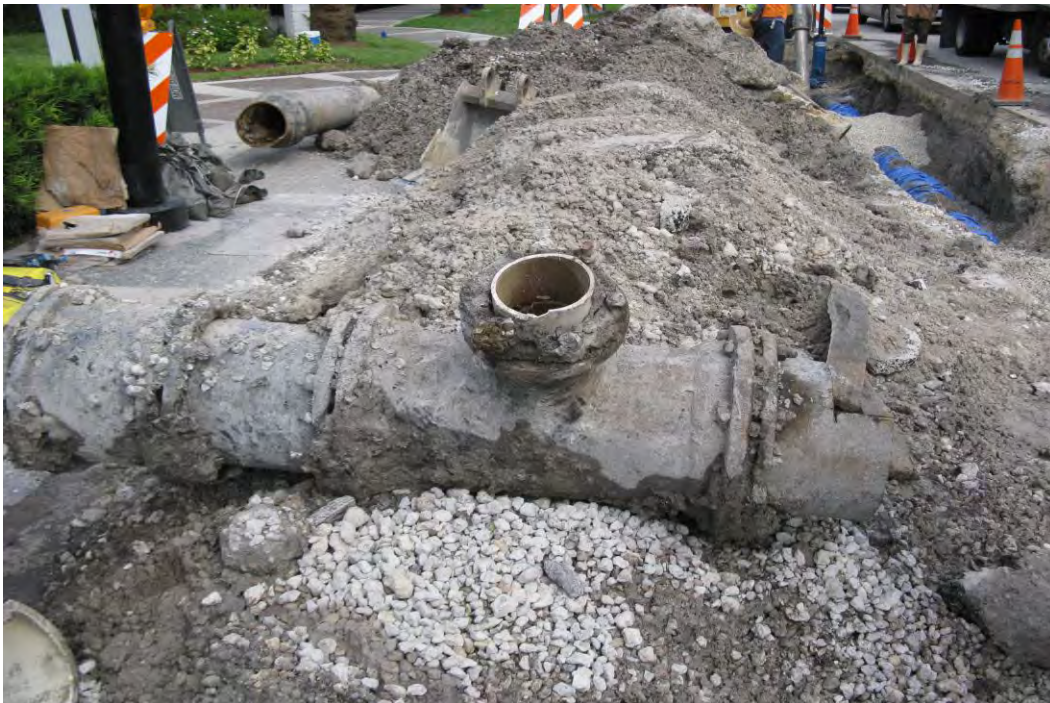
Photo 18 : Removal of existing pipe assembly.
