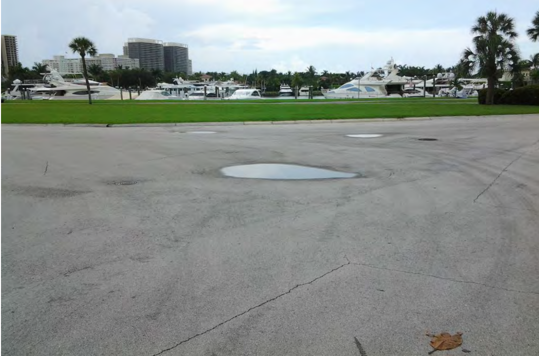
Photo 7 : Harbour Way, surface ponding and cracking, looking south.
