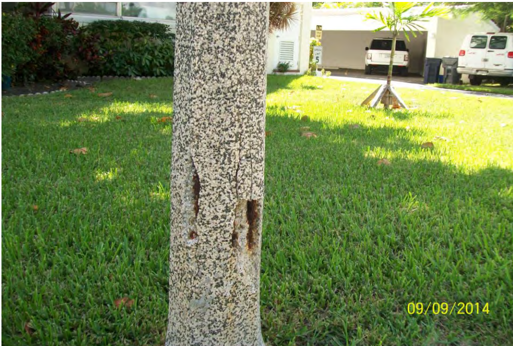
Photo 12: Damage pole base at Bal Harbour Manor and Harbour Way.
