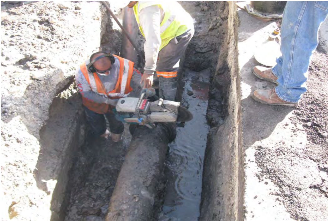
Photo 20 : Removal of existing 12" water main pipe on 96 th Street.
