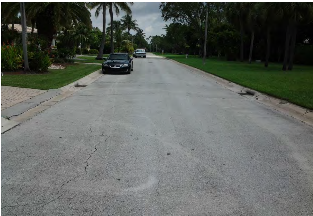
Photo 2 : Park Drive, road and curb surface cracking, looking north.
