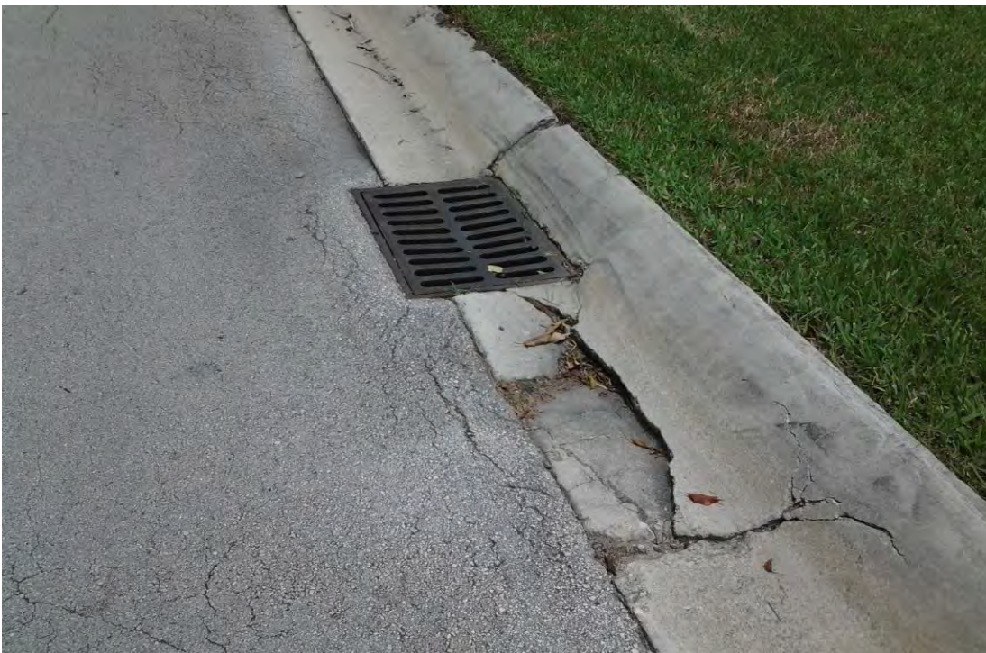
Photo 16 : Park Drive, curb failure, looking north.
