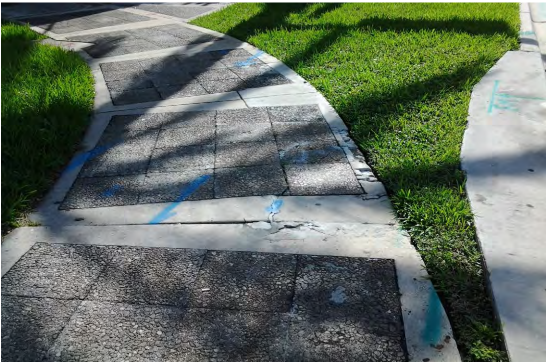
Photo 4 : Sidewalk settling, north side of road, looking east.
