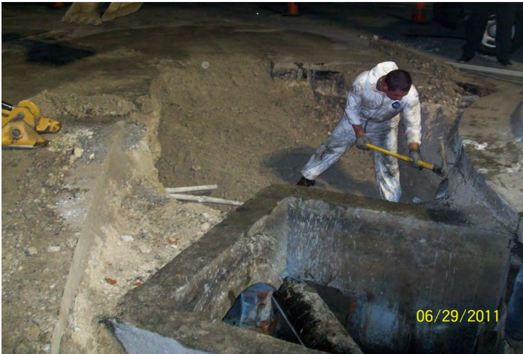
Photo 11: Sanitary Sewer Force Main repair on 96 th Street.
