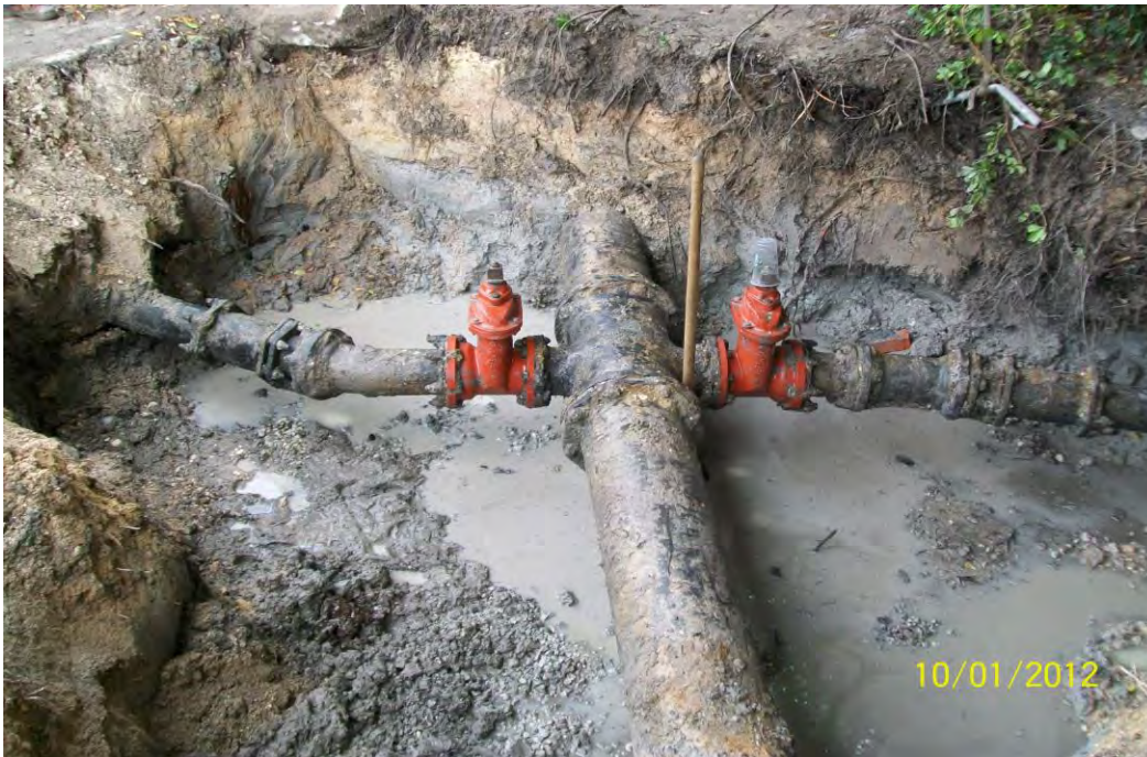
Photo 5: Existing excavated water mains on Park Drive.
