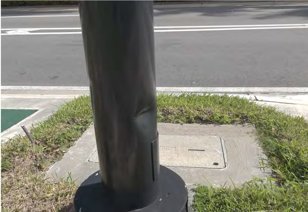
Photo 13: Existing damaged light pole.
