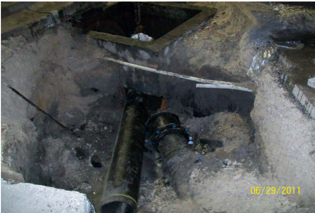
Photo 6: Force Main repair inside Drainage Conflict Structure.
