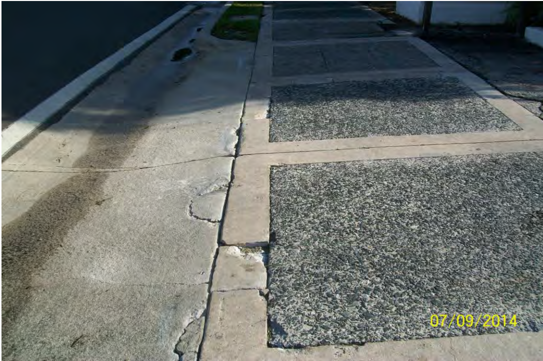
Photo 19 : Damaged walk and gutter at Carlton Terrace , looking north.
