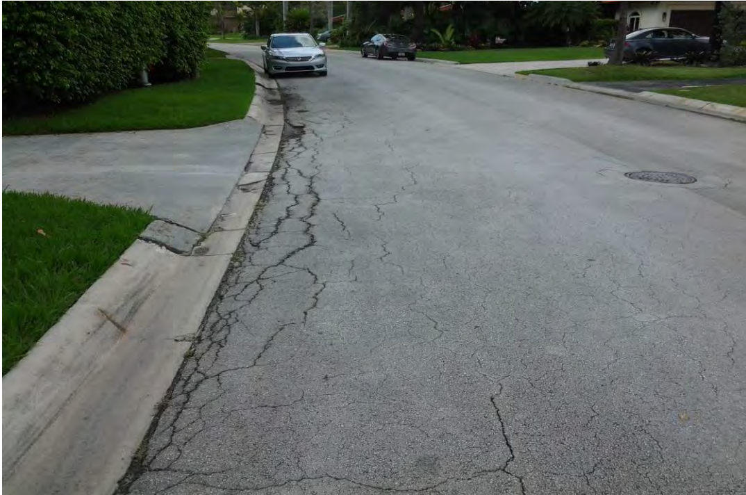
Photo 1 : Bal Cross Drive, road and curb settling, looking south.
