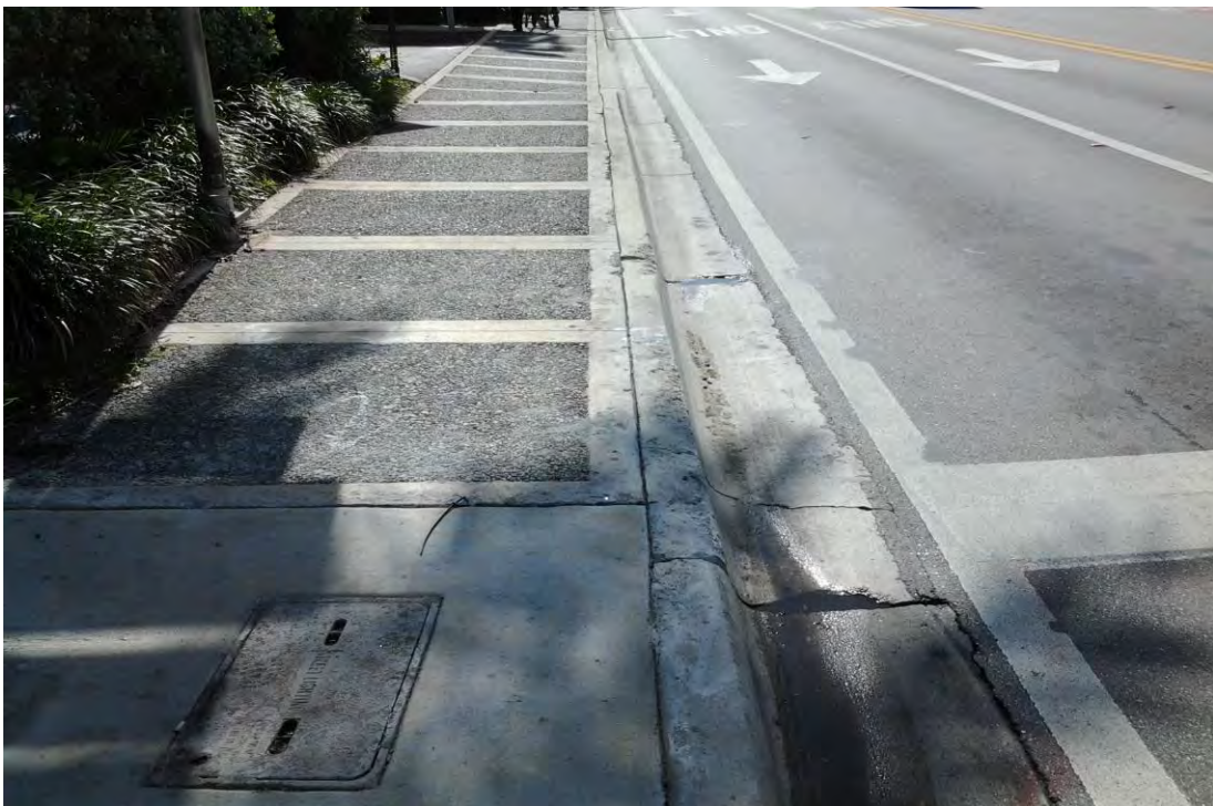
Photo 8 : Gutter separation, north side of road, looking east.
