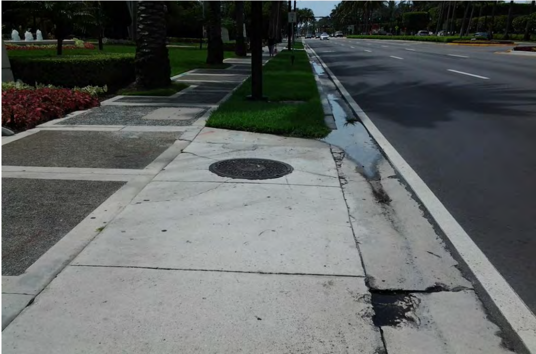
Photo 13 : Gutter failures and ponding at Bal Moral , looking south.
