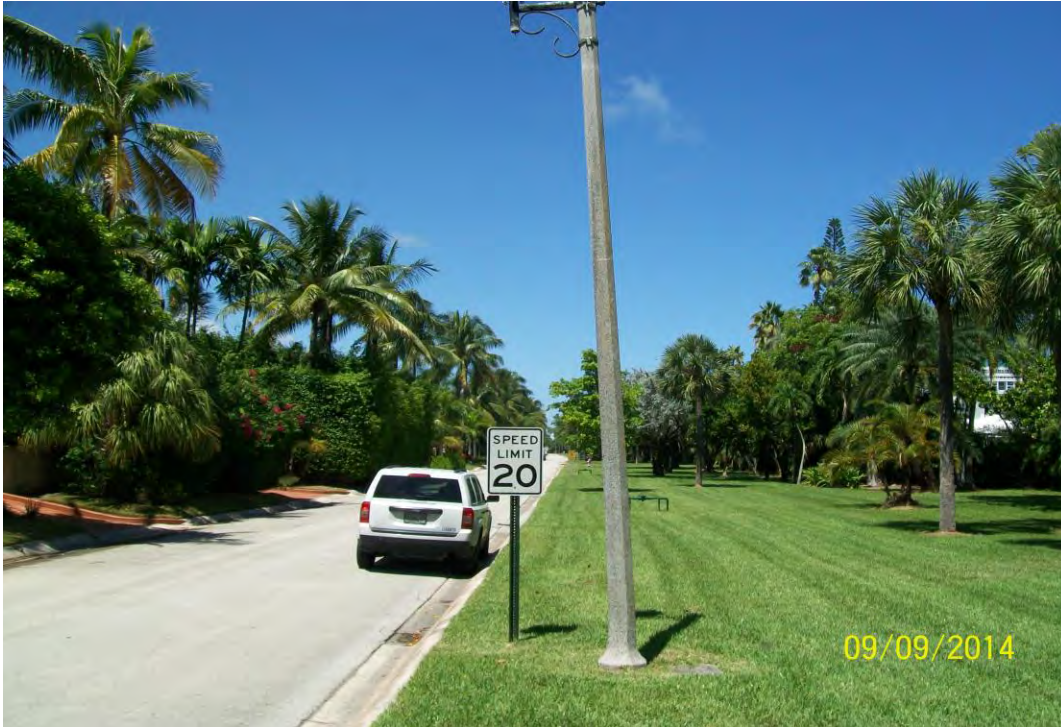
Photo 7: Leaning concrete light pole (152 Park Drive).
