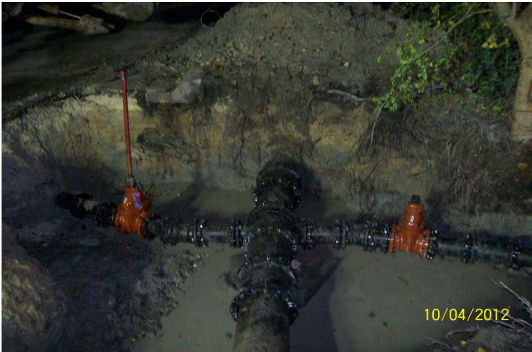
Photo 9: Completed emergency night repair of water main.
