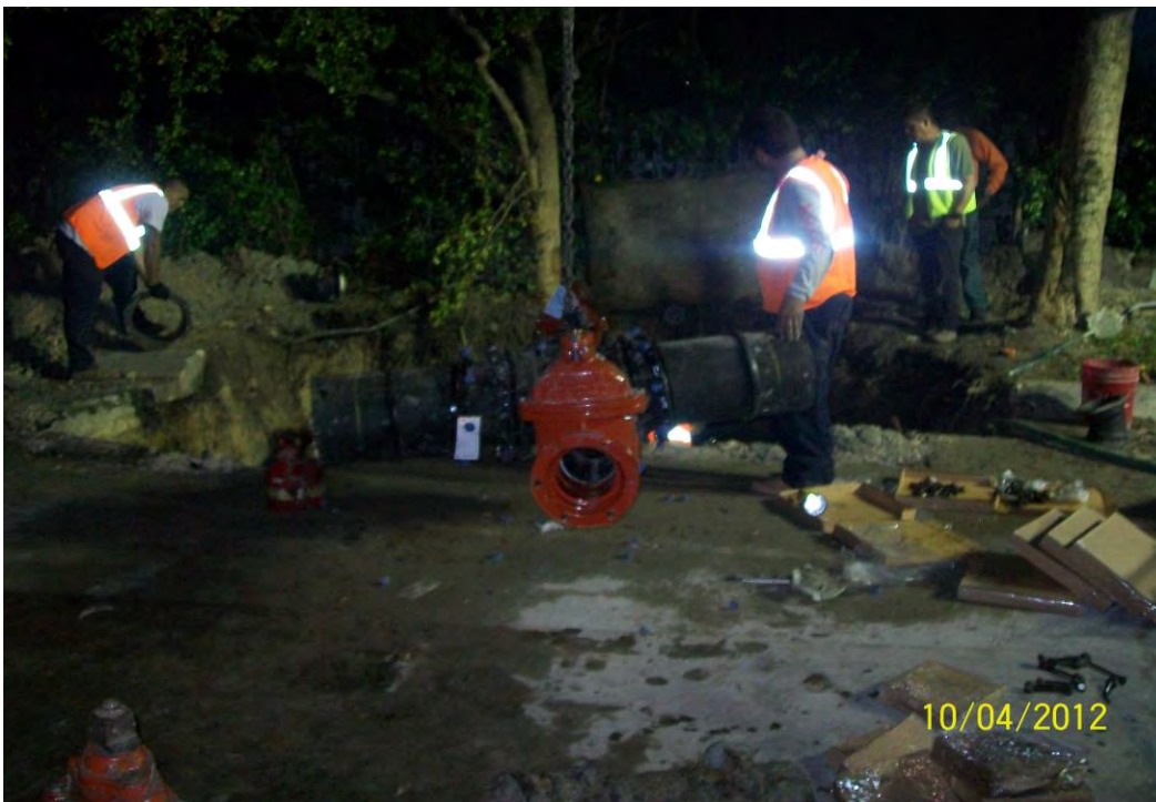
Photo 6: Night repair work on new water main assembly and fittings.
