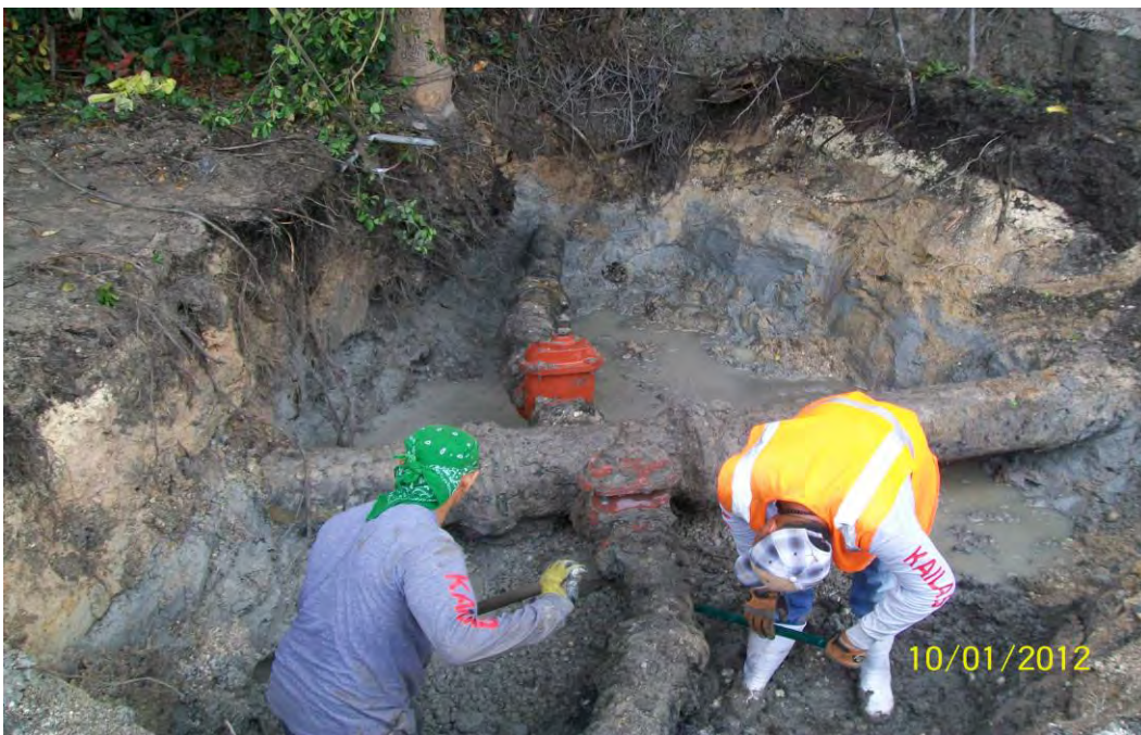
Photo 2 : Leaking Valves on 6" water main uncovered on Park Drive.
