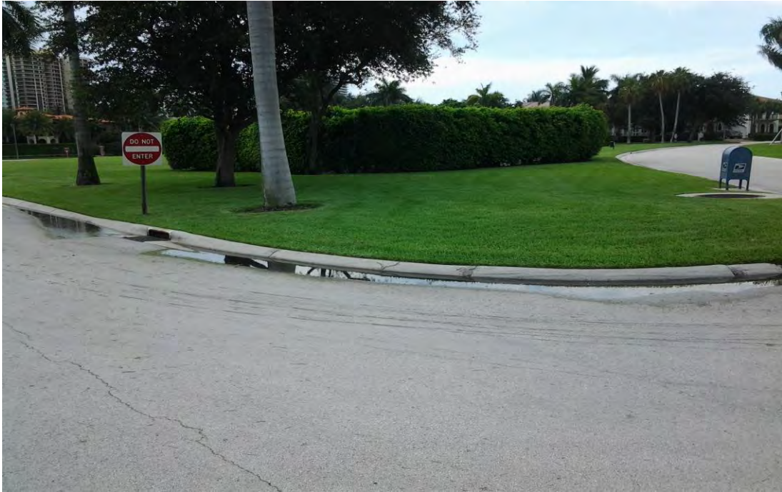
Photo 5 : Harbour Way, road settling and ponding, looking southeast.
