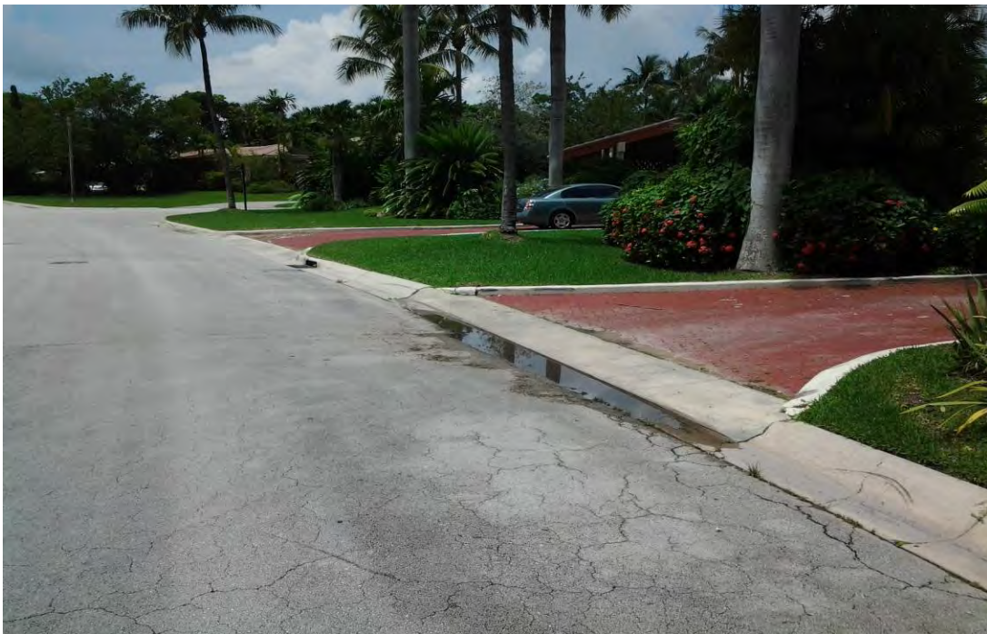
Photo 4 : Bal Cross Drive, curb settling and surface cracks, looking south.
