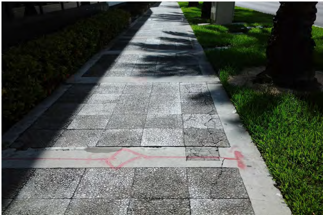
Photo 5 : Sidewalk cracking, in front of Shops , looking east.
