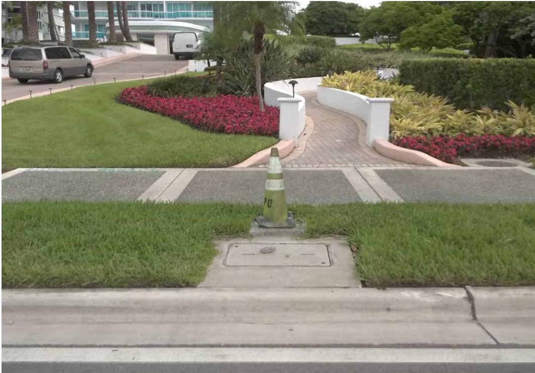
Photo 17: Missing street light behind existing pull box.
