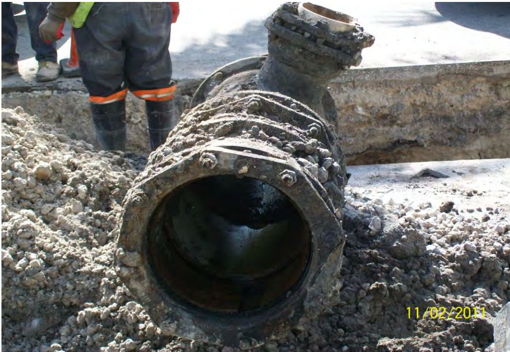
Photo 17 : Removal of existing pipe assembly.
