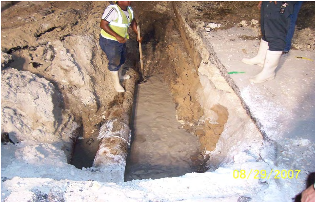
Photo 3: Sanitary Sewer Force Main repairs on Byron Avenue.
