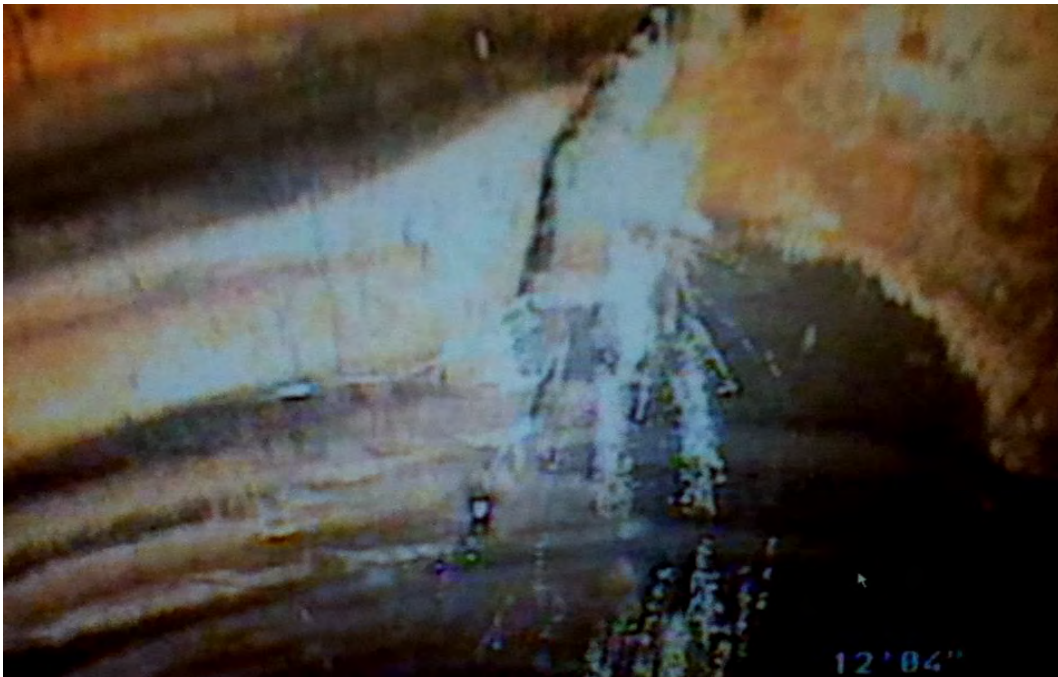
Photo 12: Longitudinal crack at top of stormwater pipe.
