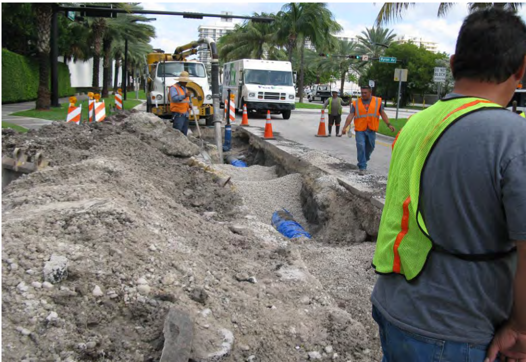
Photo 22 : Backfilled water main trench on north side of 96 th Street.
