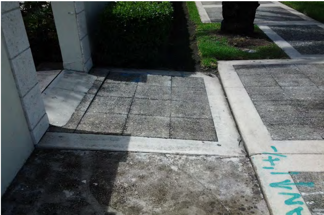
Photo 12 : Settling sidewalk at Bal Moral , looking south.
