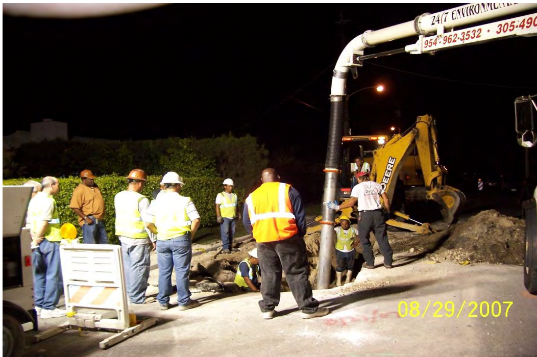
Photo 1 : Sanitary Sewer Force Main repairs on Byron Avenue.
