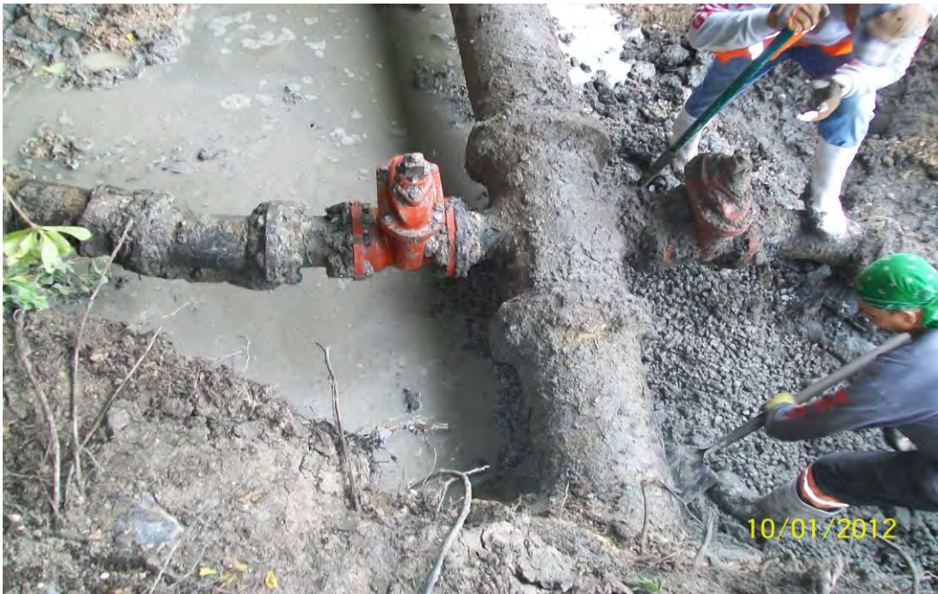
Photo 1 : Leaking Valves uncovered at Park Drive and Camden Drive.
