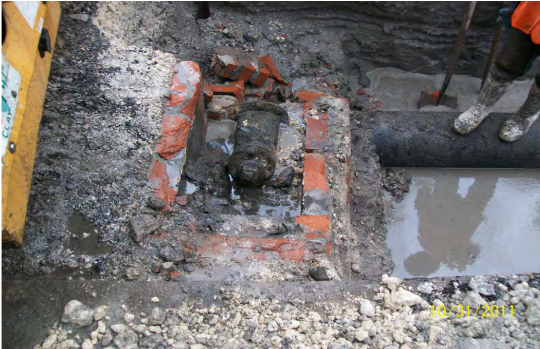
Photo 13 : Failed water main pipe uncovered on 96 th Street.
