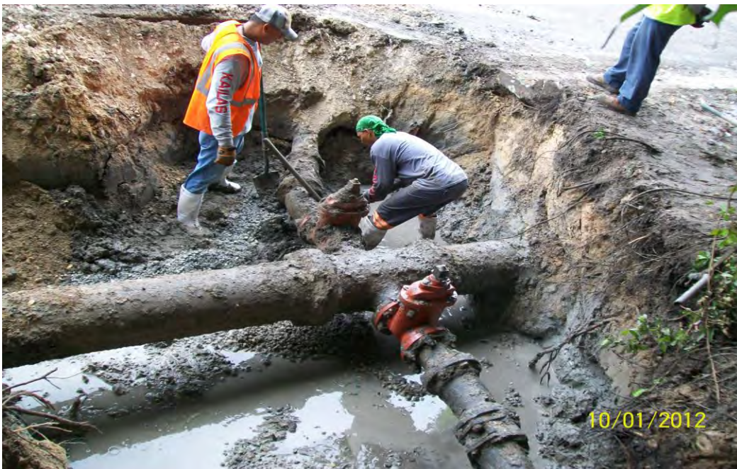
Photo 4: Exist. 6" and 12" water mains where valves were uncovered.
