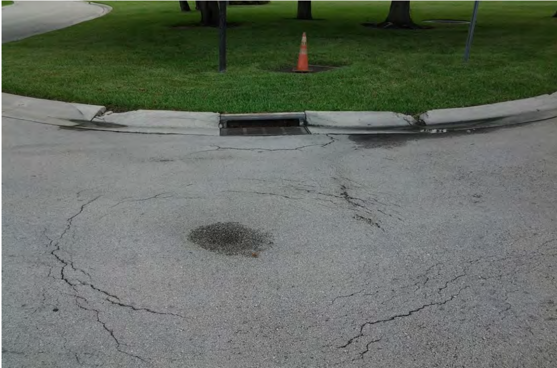
Photo 9 : Bal Bay Drive, curb and roadway settling, looking northeast.
