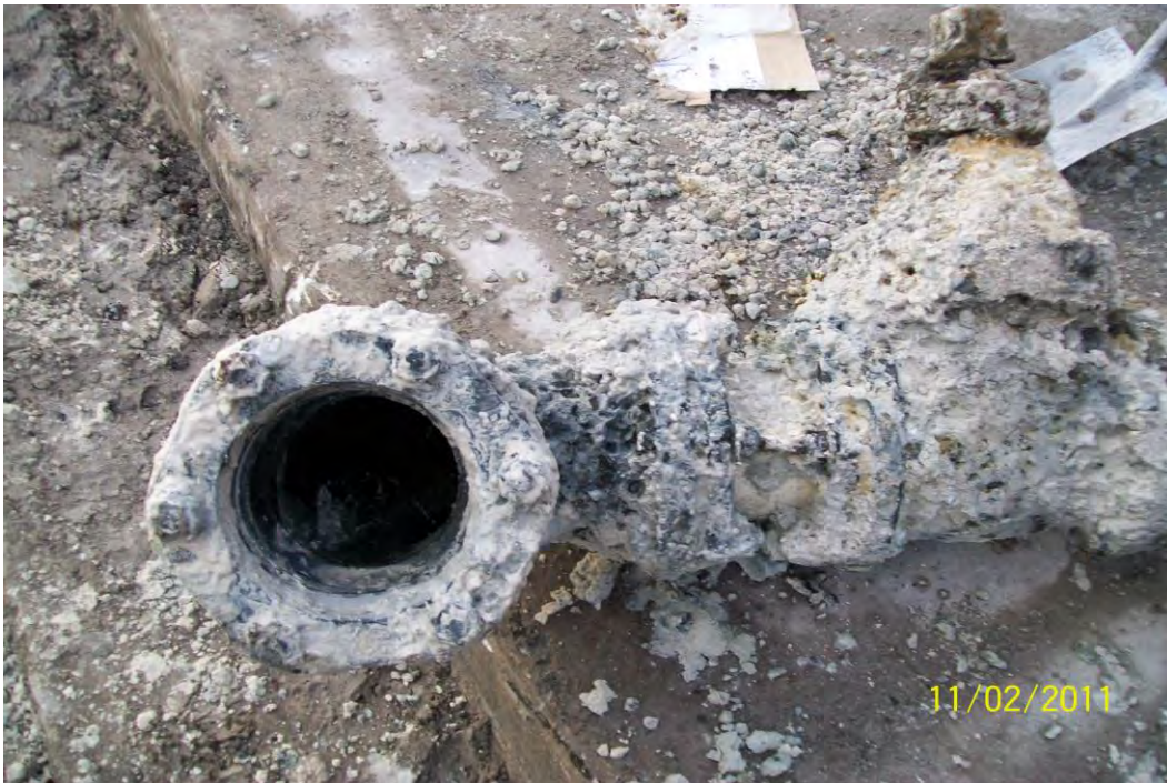
Photo 19 : Removal of existing valve assembly.
