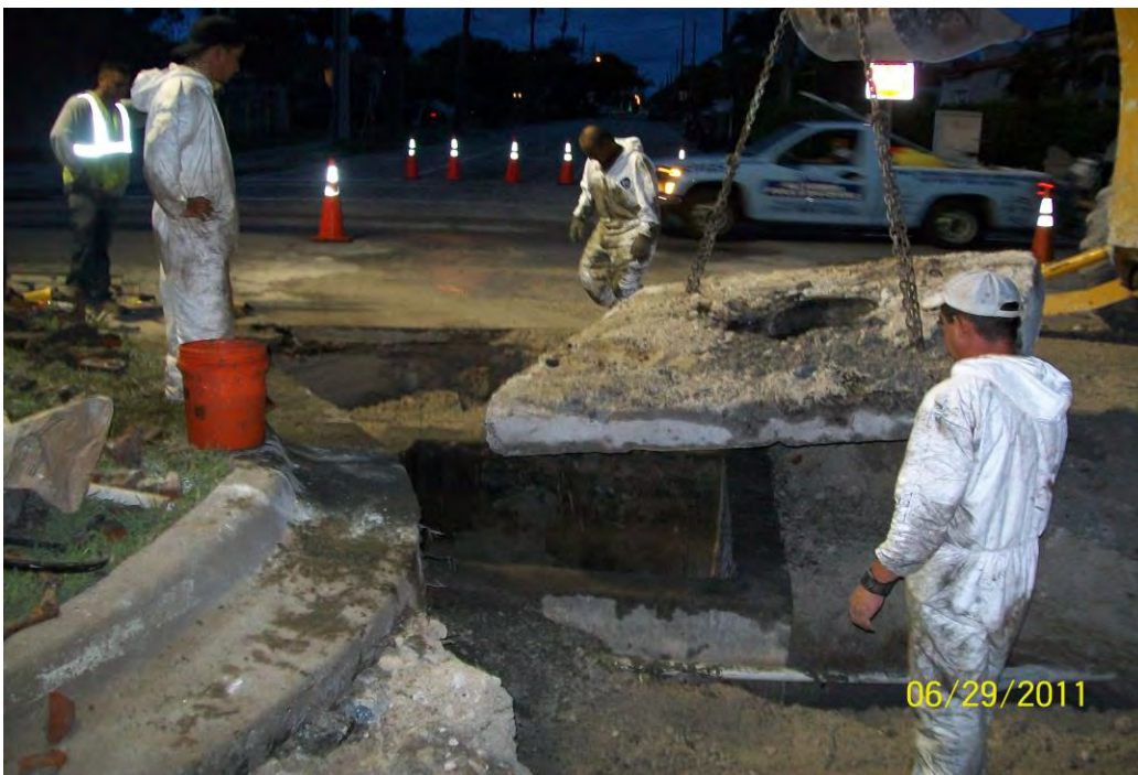
Photo 12: Sanitary Sewer Force Main repair on 96 th Street.
