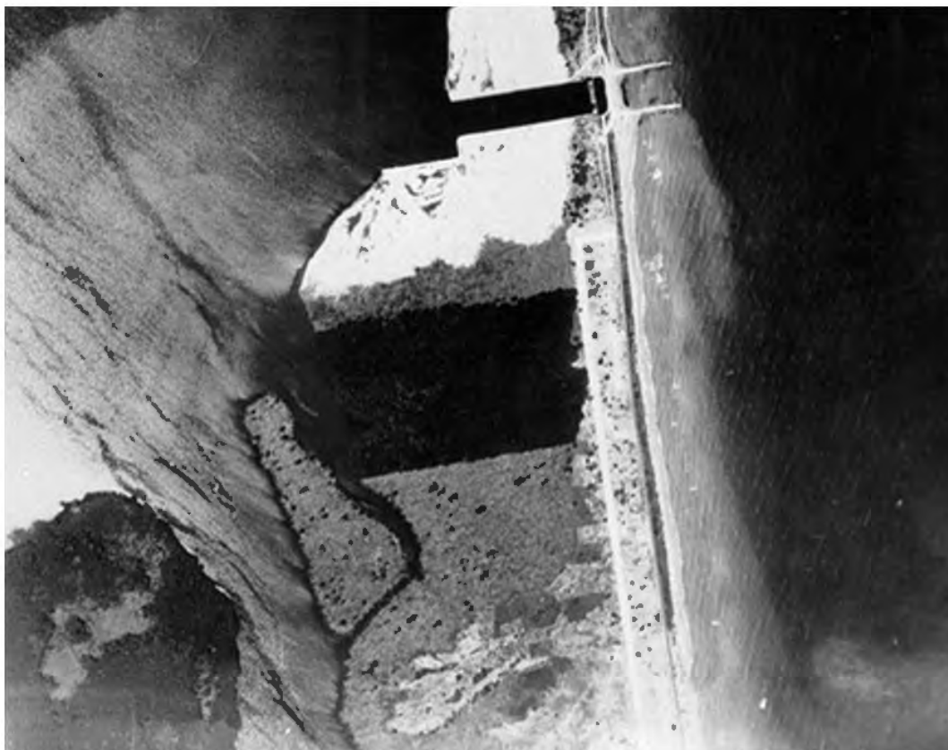
Figure 1-2: Historical Aerial (1925), Source: Miami Dade Public Library
