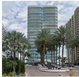
3RD BUILDING TO THE SOUTH OF SUBJECT PROPERTY
