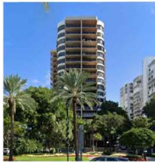
BUILDING TO THE SOUTH OF SUBJECT PROPERTY
