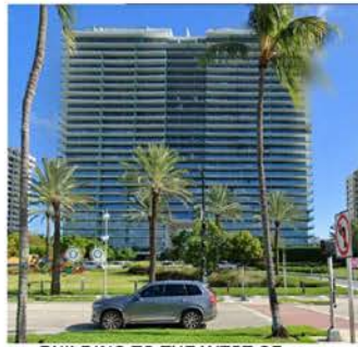
BUILDING TO THE WEST OF SUBJECT PROPERTY
