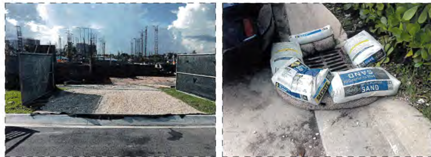
GRAVEL DRIVEWAY SAMPLE INLET / CATCH BASIN PROTECTION SAMPLE
