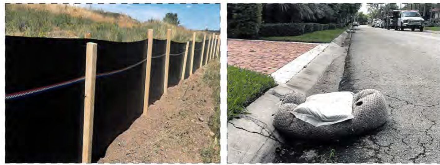
SILT FENCE SAMPLE PROPERTY LINE PROTECTION SAMPLE
