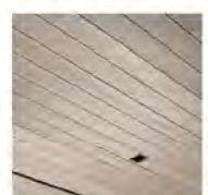
(5) WOOD CEILING, EAVES, CLADDING, & FASCIA
