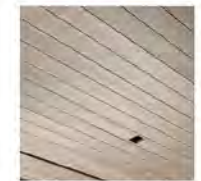
(5) WOOD CEILING, BAYS, CLADDING, & FASCIA
