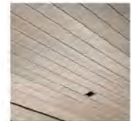
(5) WOOD CEILING, EAVES, CLADDING, & FASCIA
